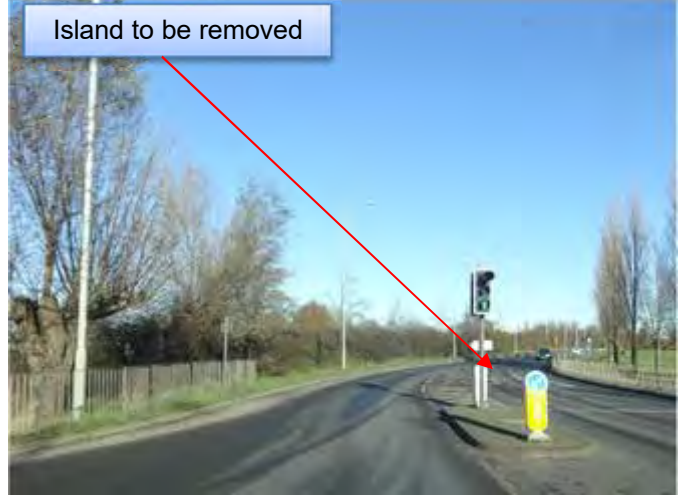
8.4.6.4. – View on junction
