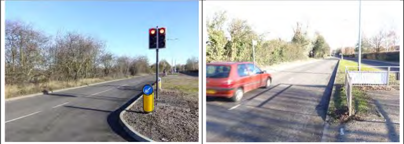
8.5.1.3. – View on junction 8.5.1.4. – View on junction
