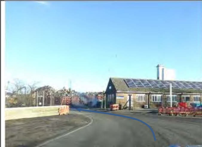
8.4.1.3. – View at crossing
